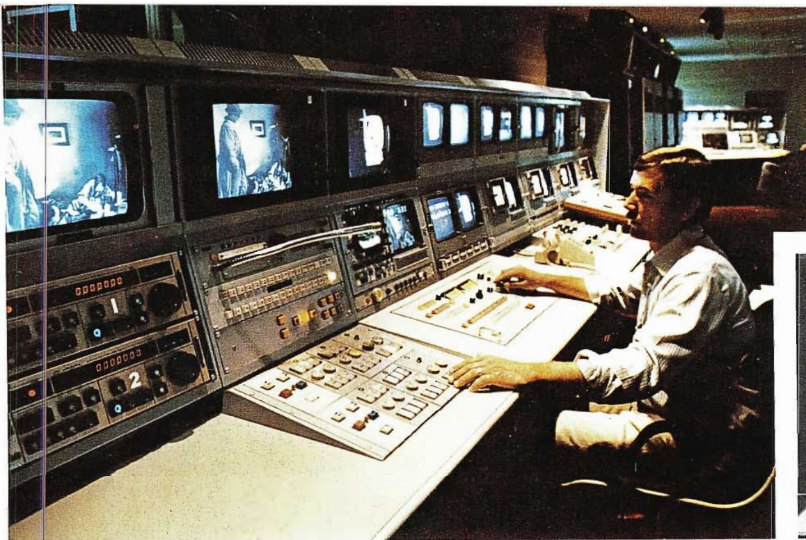
Master Control Console (left and below) provides complete machine controls for operator, and a direct look-in at the 110 kW transmitter operation.
