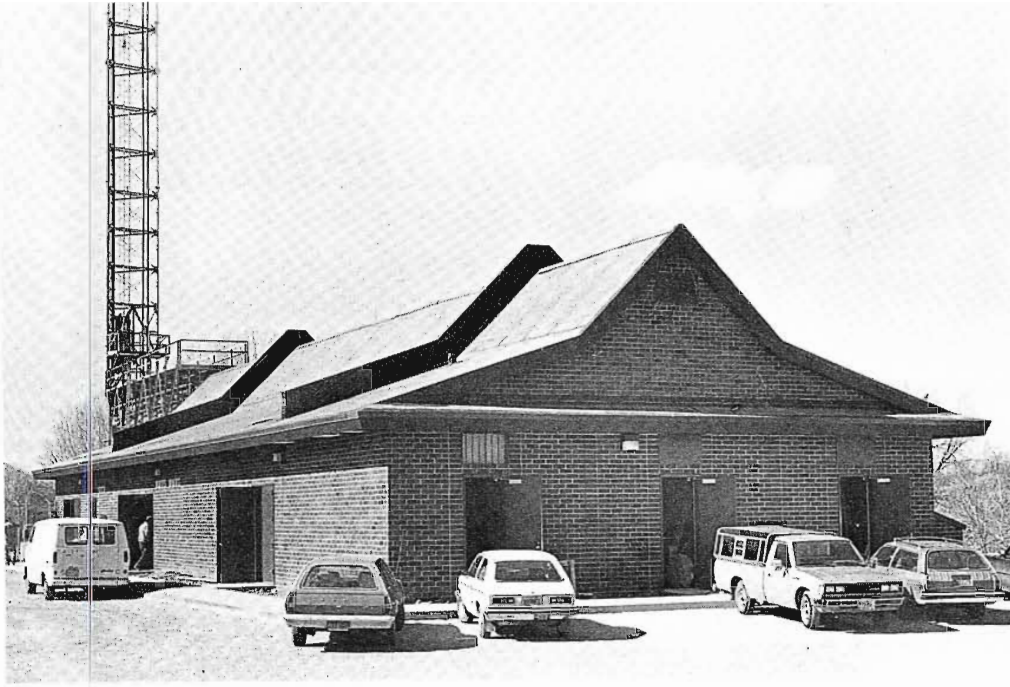
Transmitter building is currently shared by three TV transmitters and an FM transmitter, with additional space available for another FM transmitter operation.
