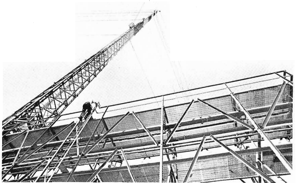
Heavy-duty catwalk from transmitter building to tower protects transmission line from ice damage.
