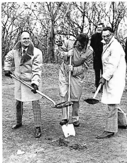
Breaking ground for the new tower on March 31, 1980 are (left to right) Harold Wagner, Chief Engineer for WMVS/WMVT; Joseph Loughlin (then General Manager of WVTV), and Bill Witt, Director of Engineering for WVTV.
